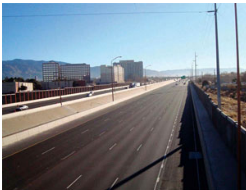
Photo: Matthew Nighbert / Gannett Fleming West
